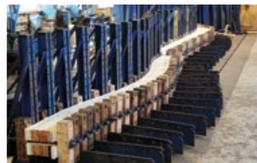
CURVED LAMINATED BEAM IN PRESSING BED
