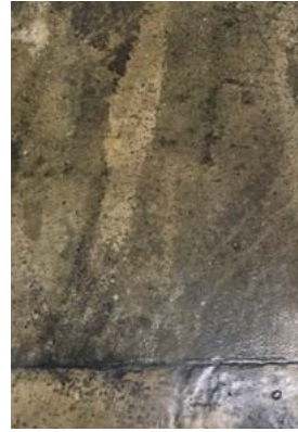
Fig. 4: Floor sealed with resin, slight reflection
