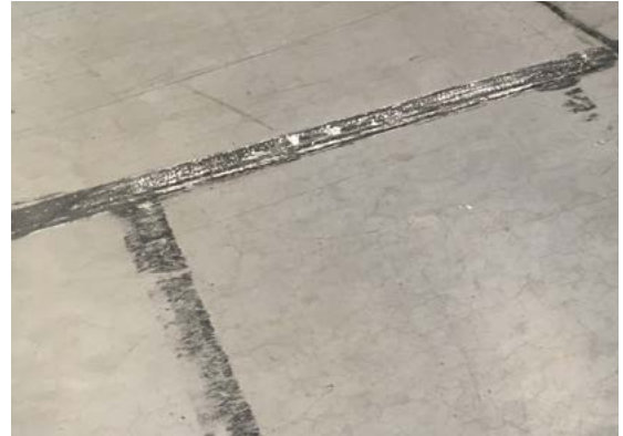
Fig. 1: Abrasion on floor markings
